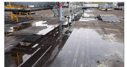
Roof Area B – Partial overview of roof area; ponding water over primary east/west corridor
